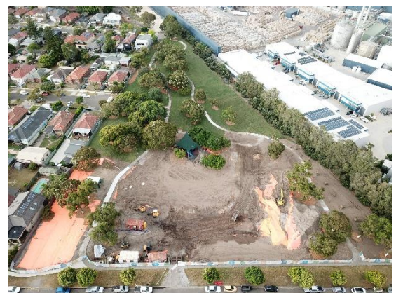
Figure 1: aerial photo of capping works at Purcell Park 2020
